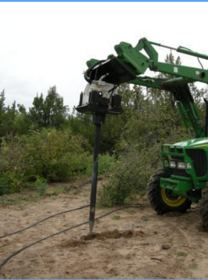
Hydraulic compactor with stinger (3.5-inch diameter) attached to the loader of a 65-hp farm tractor
