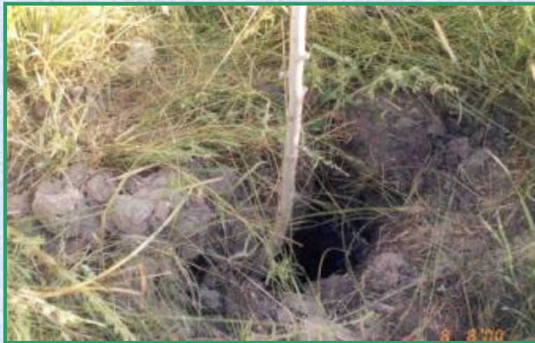
Improper backfilling
