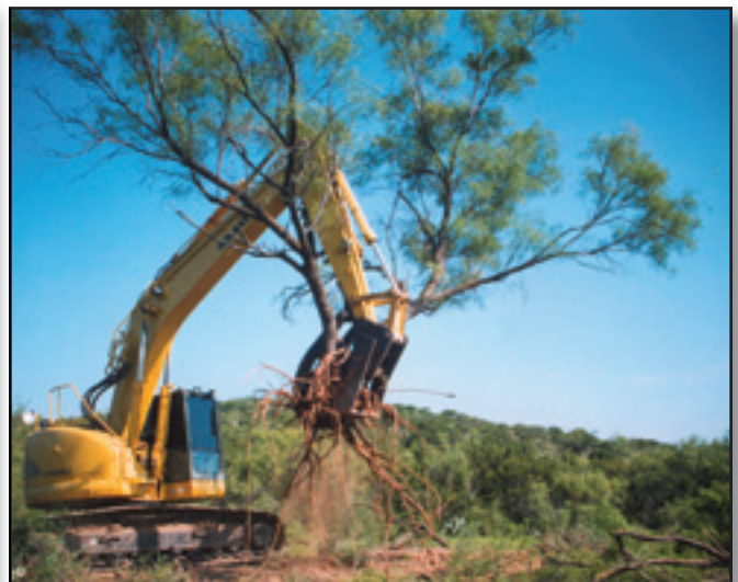
Figure 18b—Boss Reclamation equipment at work (Photo courtesy of Boss Reclamation, LLC).
