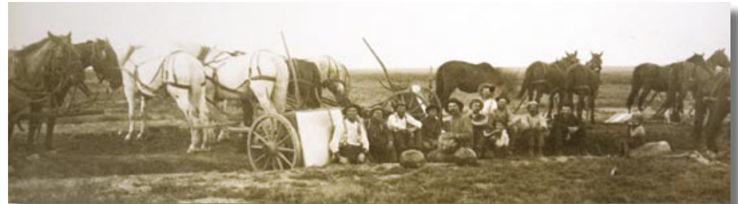
Workers take a break from digging a ditch near the Pleasant Valley School in Greeley. Most early settlers possessed no experience or equipment for building irrigation canals, and ended up using their own teams, plows, pick-axes and shovels.
