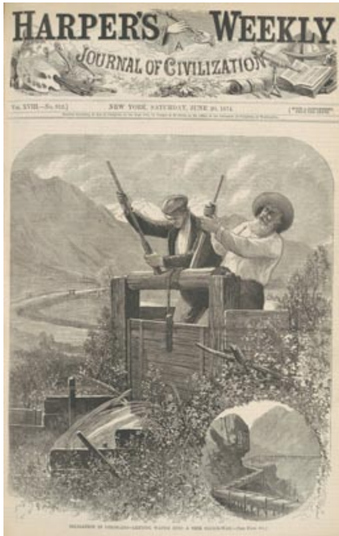
Harper's Weekly was one of the most popular illustrated newspapers of the 1800s. In this 1874 edition, the Union Colony and Colorado irrigation made the front page in an engraving captioned "letting water into a side sluice-way" in reference to what are now called "headgates."
