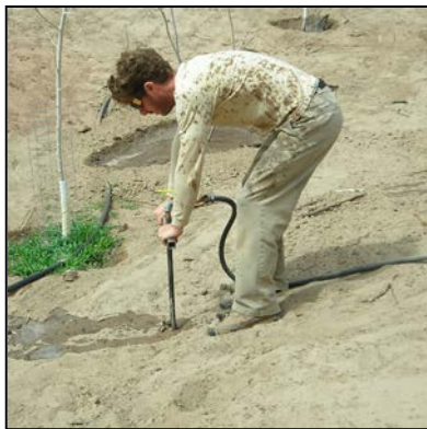
The water jet stinger works well in sandy sites to deeply plant poles that will not wash out in flood events
