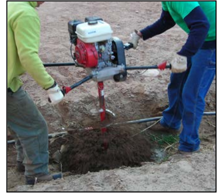
A two man auger can be used in areas where equipment cannot reach to deep plant cottonwoods and other riparian species
