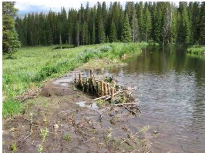
Figure 63: A PLWW was constructed on one repaired dam to temporarily fortify a nick point while we were waiting for beaver to reoccupy the site
