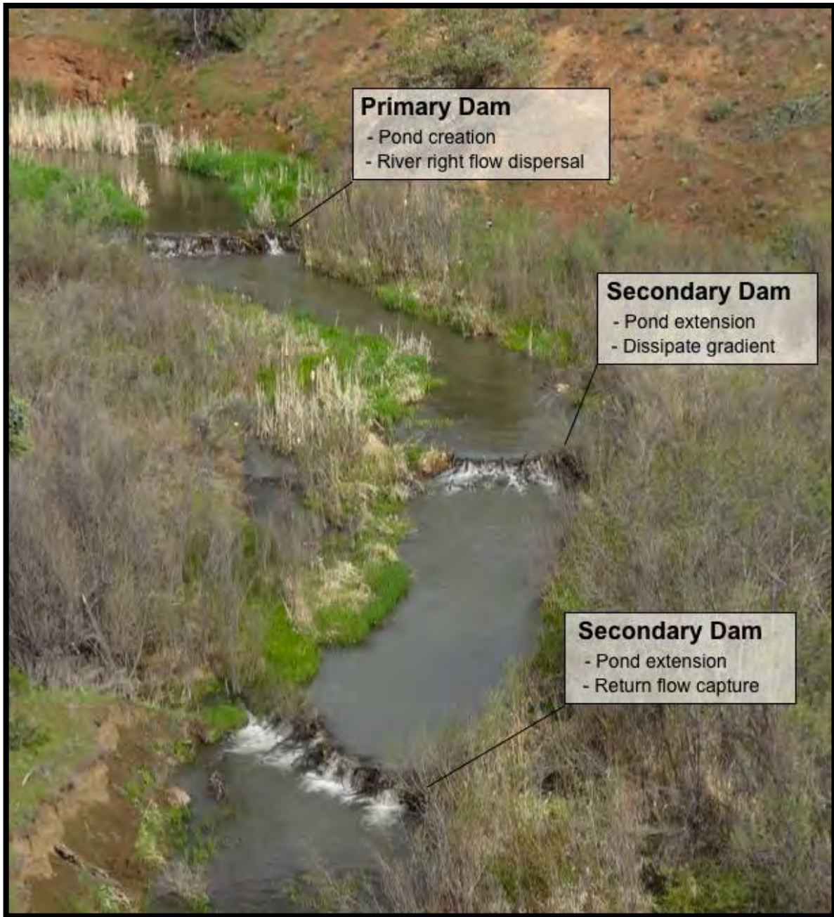
Figure 29: Example of a sequence of beaver dam analogues on Bridge Creek, in Oregon. The primary dam is a reinforced existing dam originally built by beaver, while the secondary dams are post lines with wicker weaves that self-sealed with sediment and organic material. The primary dam has remained stable for more than 5 years and has created extensive flooded wetlands on river right. The secondary dams create pool habitat, dissipate energy, capture return flow, and raise water levels, which reduce the potential for headcutting on return flow side channels, while also increasing the floodplain inundation period. (Photograph and graphics by N. Weber).
