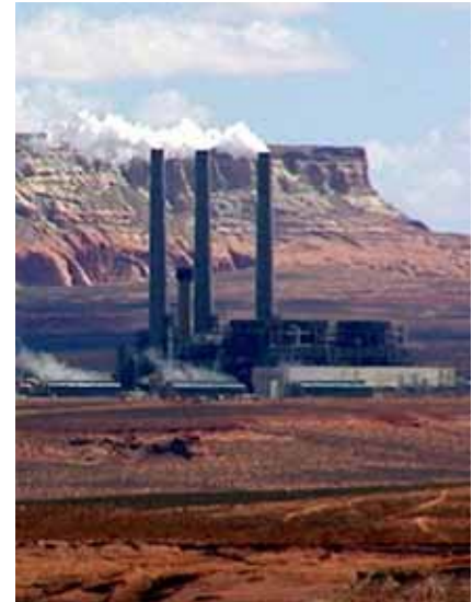
Navajo Power Plant
