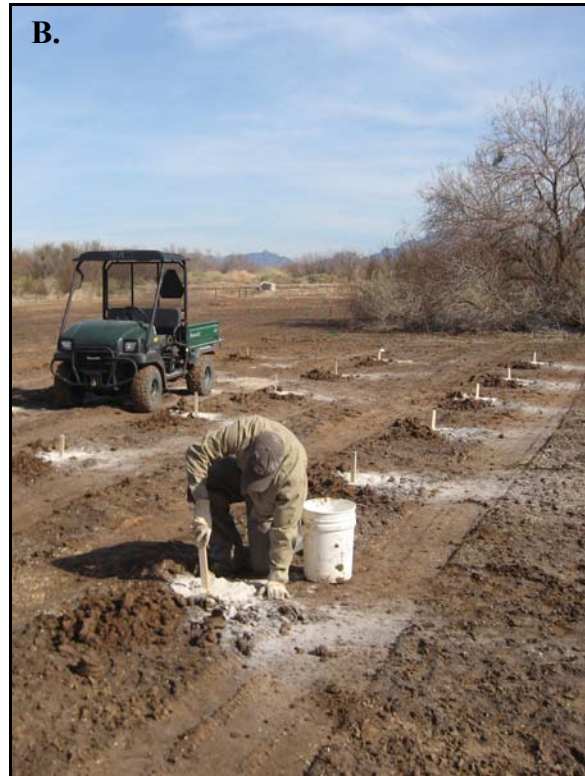
Figure 10. Drill rig used to auger holes at the study site (Image A), and backfilling of holes with zeolite (Image B).
