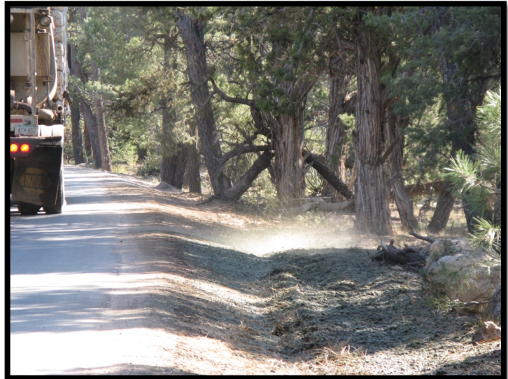
Hydromulch slurry being applied by truck mounted high velocity spray gun.
