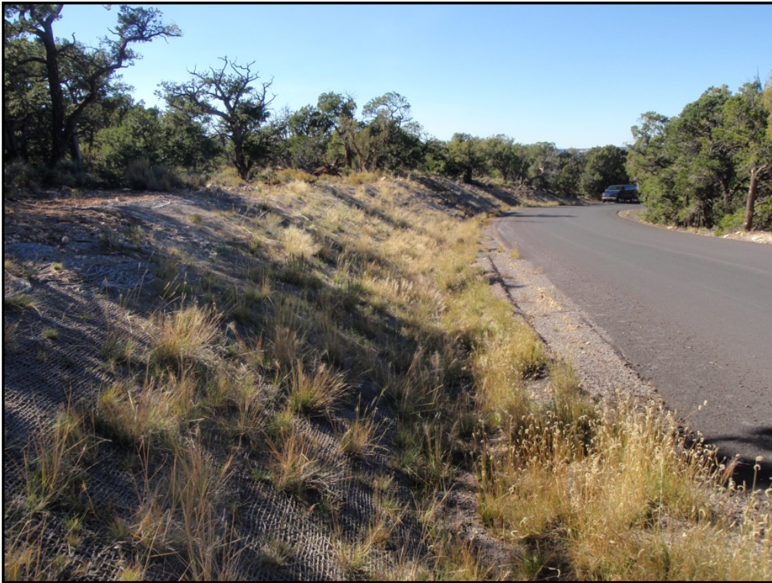
Pima Point slope with coconut fiber coir mat in October 2008 (upper) and October 2011 (lower).
