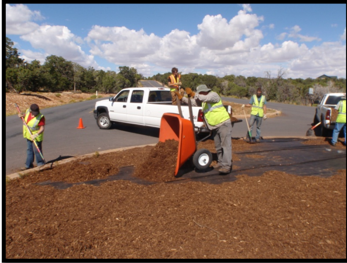
Staff spreading chip/shred mulch at a construction site.
