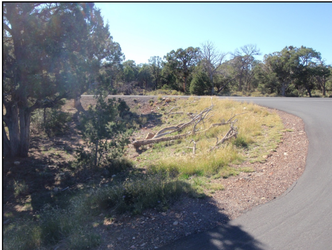
Powell Point, west exit, in October 2008 (upper) immediately following planting, and in October 2011 (lower). This slope was planted with three species of grass plugs approximately 12 to 18 inches apart and was not seeded.
