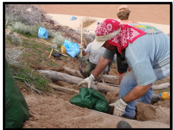
Backfilling with sand in sand ladder construction. Owl Eyes, February 2009.
