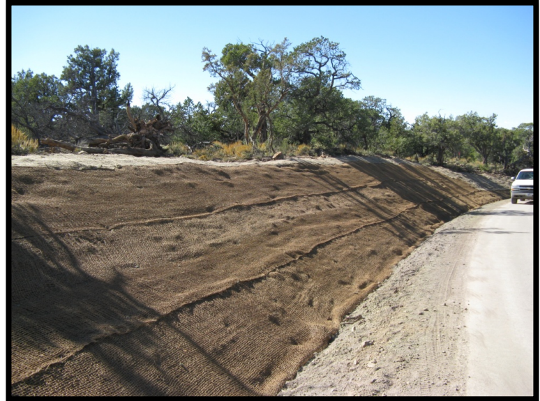
A 3:1 and greater slope immediately after being covered with coconut coir erosion control blankets. This slope was also seeded and hydromulched with the same seed mix, on the same day as the slope in the photo above.
