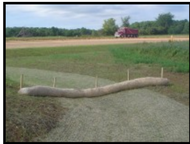
Aspen fiber (Curlex) erosion control wattles installed in a drainage.
