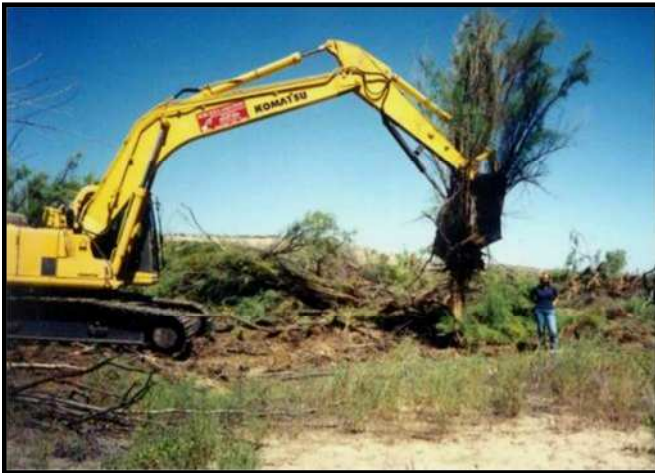
Figure 3.4 Root crown extraction using tracked excavator.
