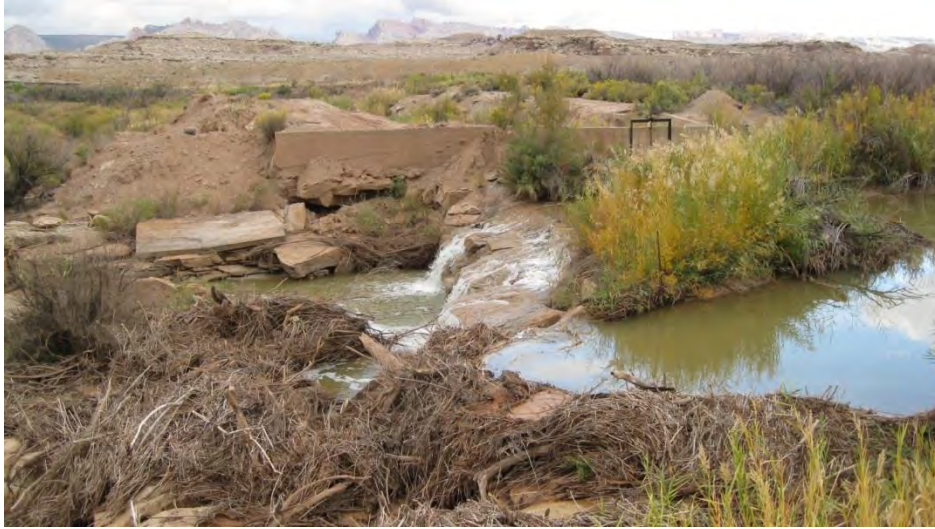
Figure 5. Picture of Hatt's Ranch diversion dam, which is a barrier to upstream fish movement. The dam is located on bedrock and was constructed in its current location in the early 1950s. Photo by B. Laub on October 12, 2012 at a flow of 18 cfs.
