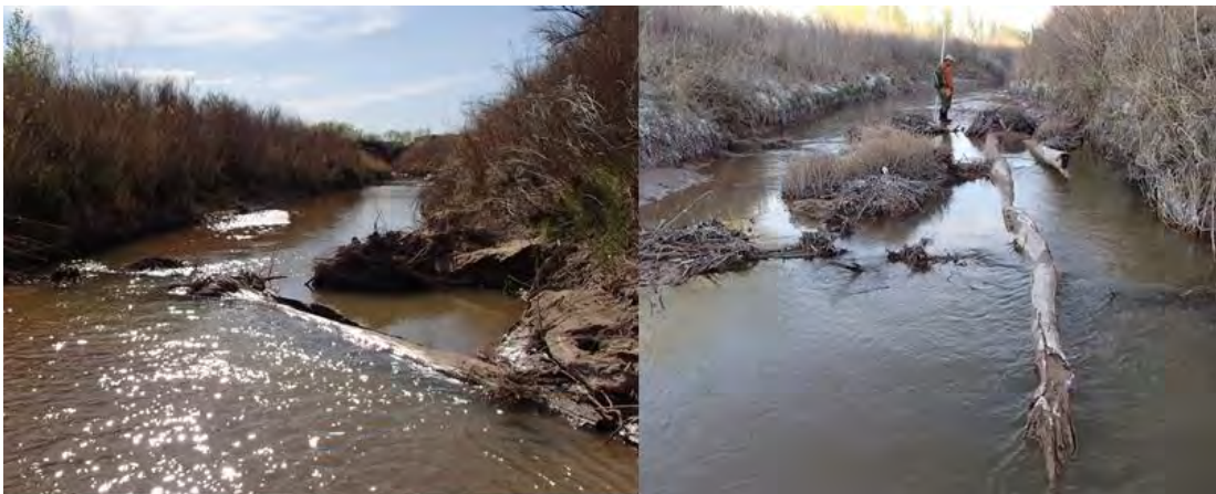
Figure 28. Pictures showing the intended effects of large wood additions to the channel. In both pictures, large logs and other wood accumulations in the channel create variations in flow and depth in an otherwise straight, generally uniform channel.
