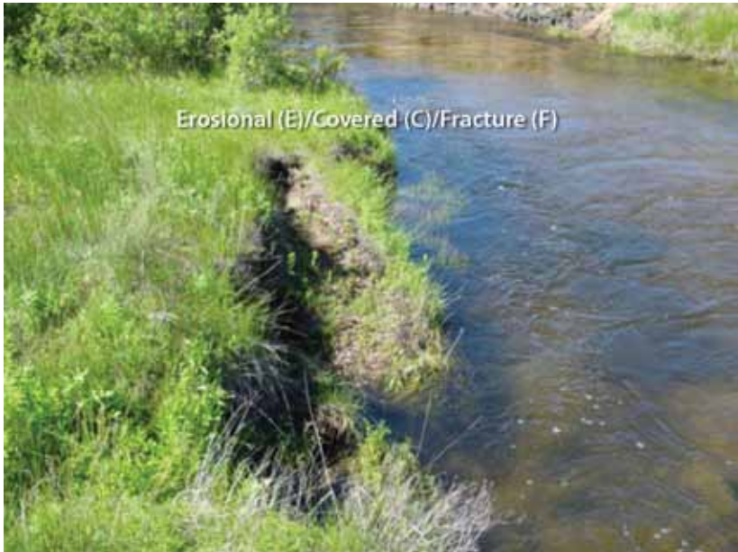
Figure E4. This large fracture has at least 50 percent vegetation cover and is thus recorded as erosional (E), covered (C), and fracture (F).
