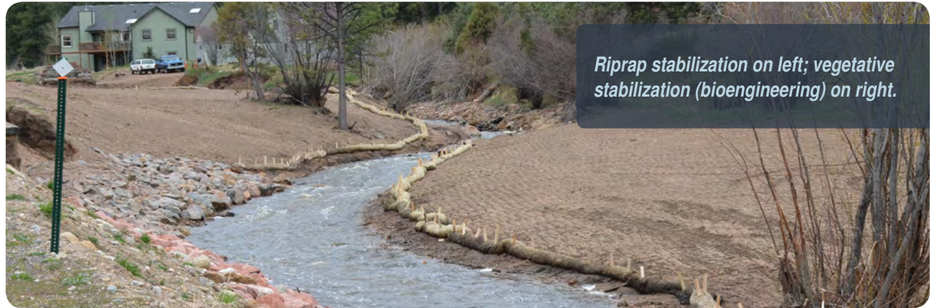
Boulder toe bank stabilization
