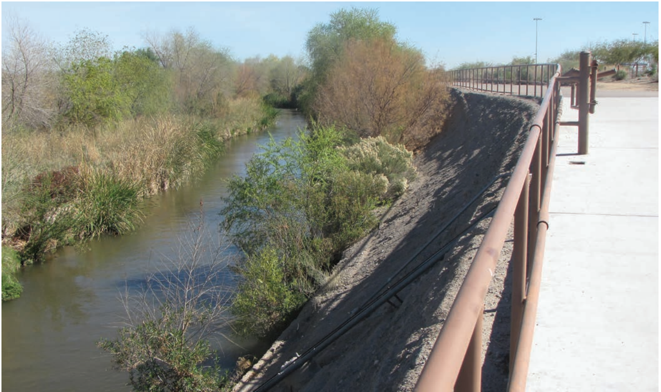
Figure 20 —Riparian habitat: effluent-dominated reach of Santa Cruz River in Tucson, historically dry, currently wet. Note narrow width of riparian vegetation and soil cement bank. Photo by author.
