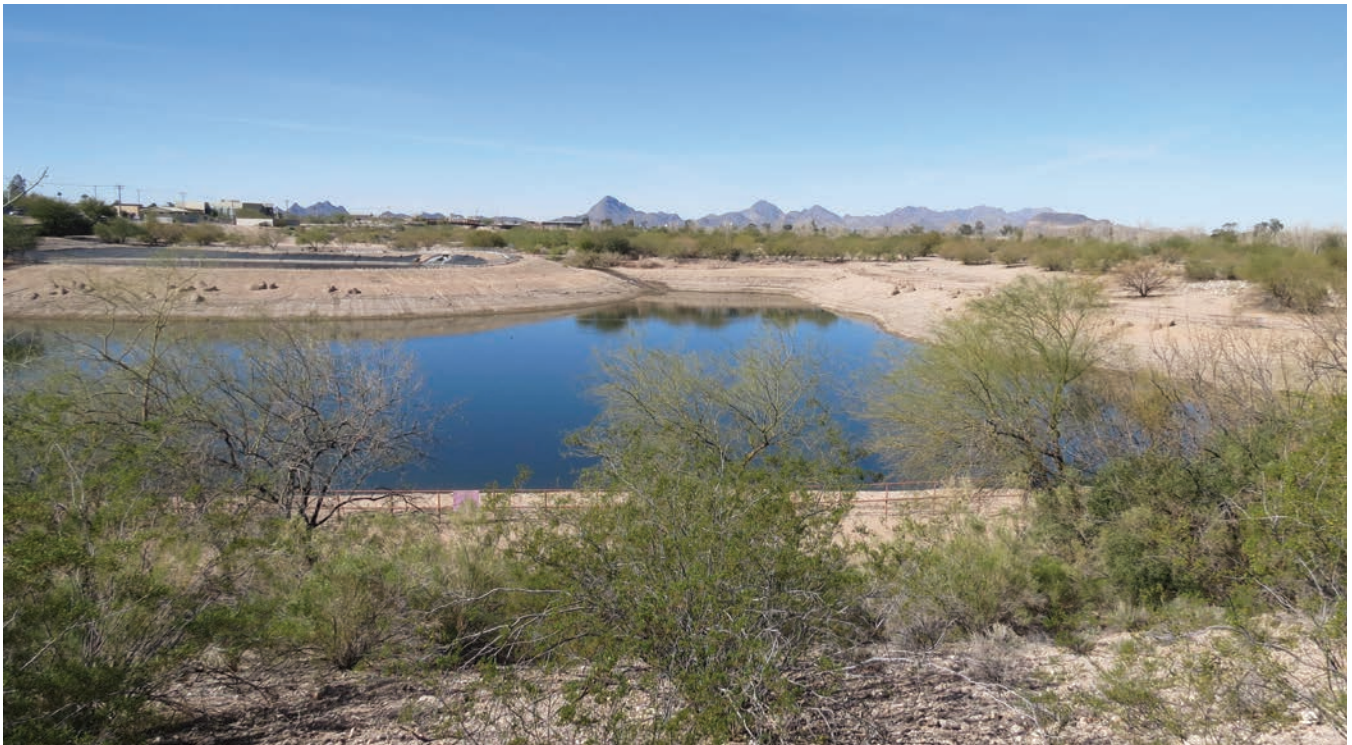
Figure 23 —Riparian habitat: Kino Environmental Restoration Project, deep pond and vegetation, February 2014. The pond was created primarily a receptacle for stormwater runoff from the upstream urban area, and is managed, in part, to provide wildlife habitat and as a recreational amenity. Its design and management allow for rapid filling following storm events and minimization of mosquito habitat. Photo by author.
