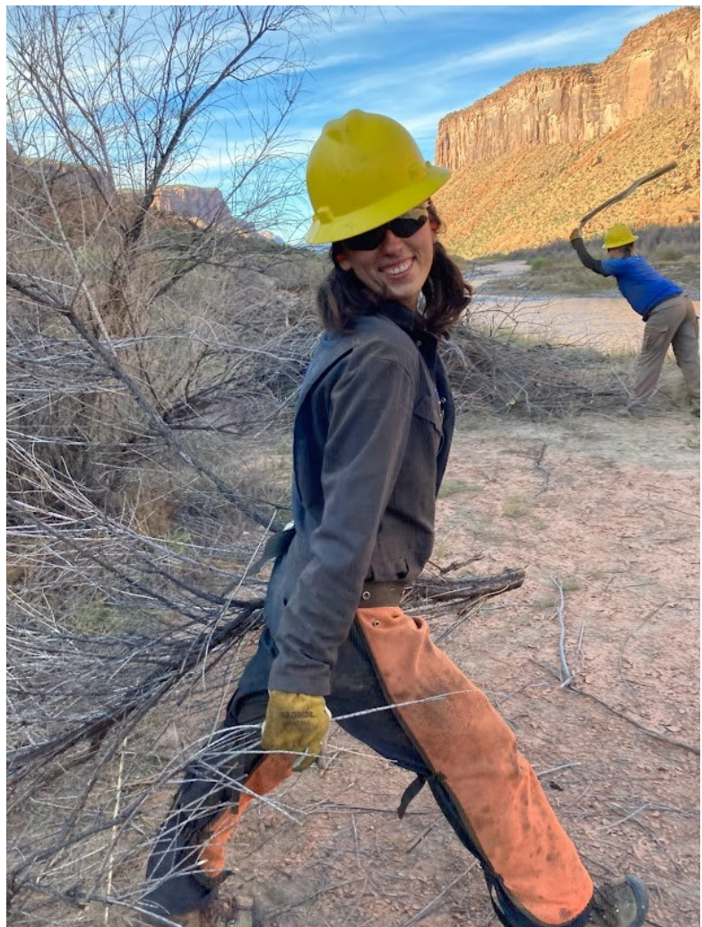
WCCC crew members dragging and piling cut tamarisk. Photo credit: WCCC
