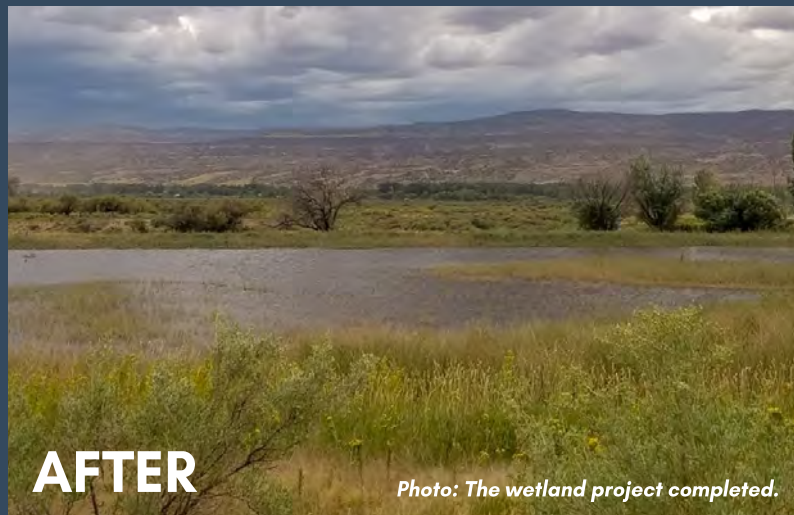
Photo: The wetland project, mid-construction, with the wetland embankment completed.
