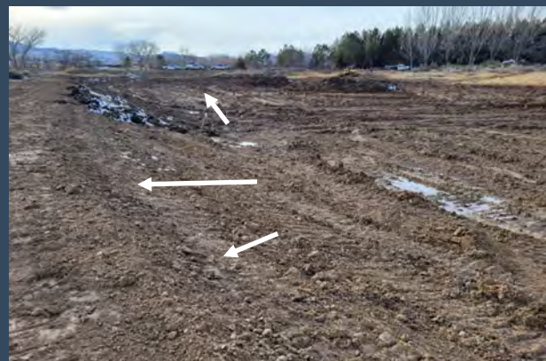
Photo: The wetland project, mid-construction, with the wetland embankment completed (denoted by arrows)
