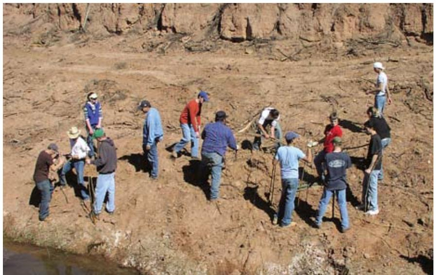
The main objective of this long-term effort is to reduce the amount of sediment transported into the Rio Grande, working throughout the headwater regions of the five main drainages of the Abó Arroyo to protect banklines, reduce runoff velocity, induce stream meandering, and re-establish healthy riparian and wetland areas. Nearly one-half of the river's mileage has been treated under the plan.
